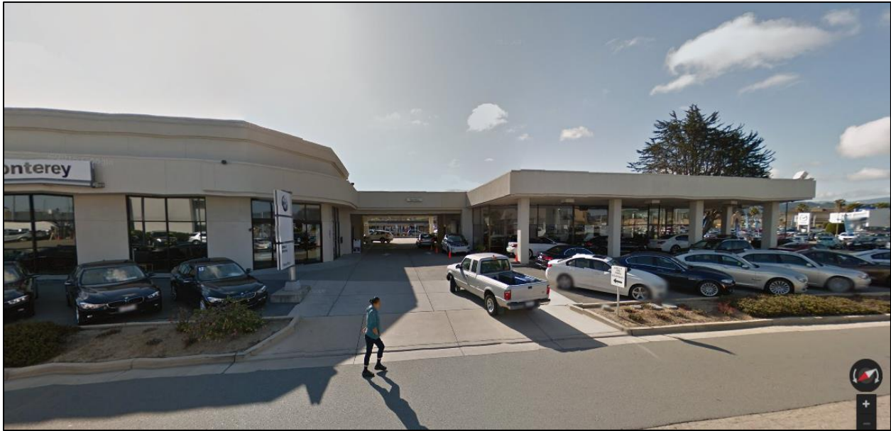
View of Service Entrance from The Mall
