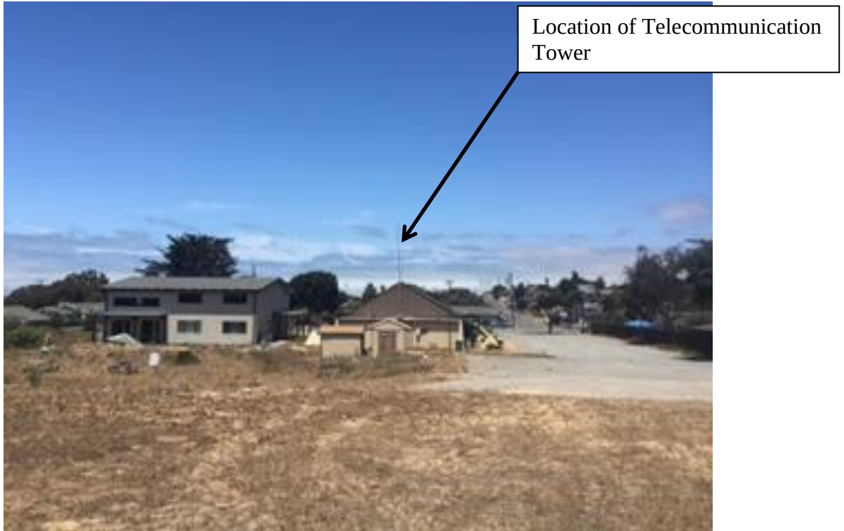
View from rear of site looking north
