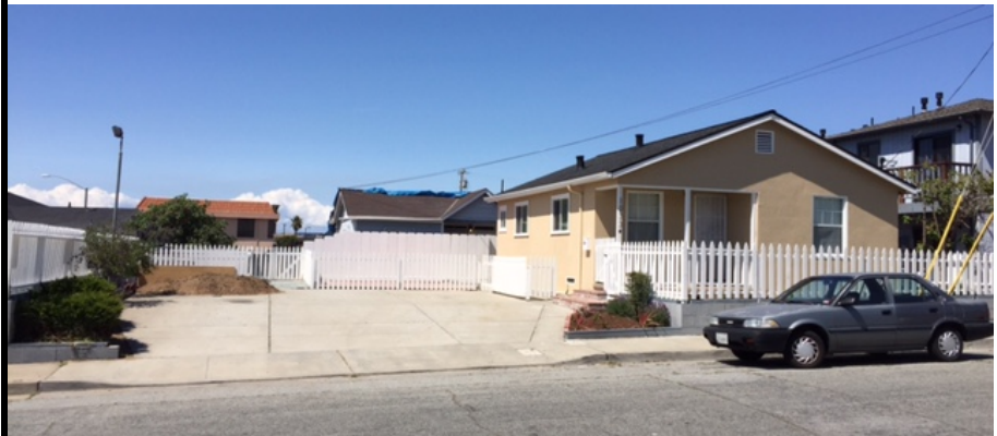
Unit A Property Frontage on Olympia Avenue
