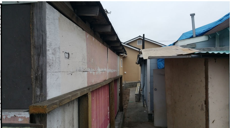
Existing garage from alley fence
