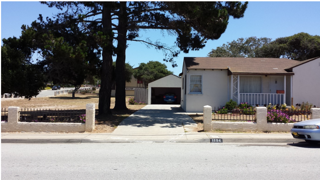
View of front showing parsonage and garage from Noche Buena Street
