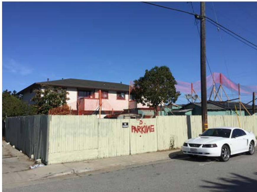
View from Terrace Street looking to the West
