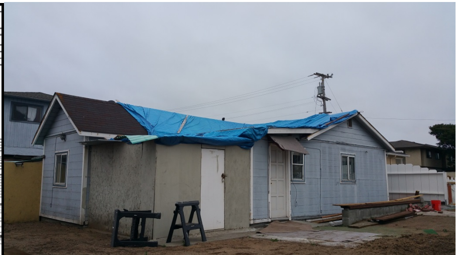
Unit B-Location of rear addition (demo existing non-permitted addition)
