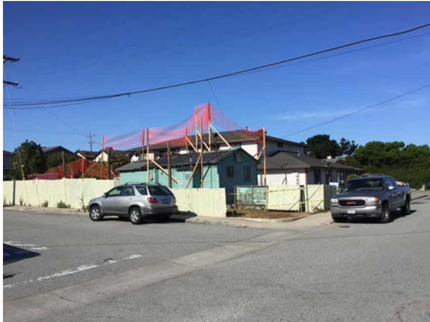
View from Clementina Avenue and Terrace Street looking southwest
