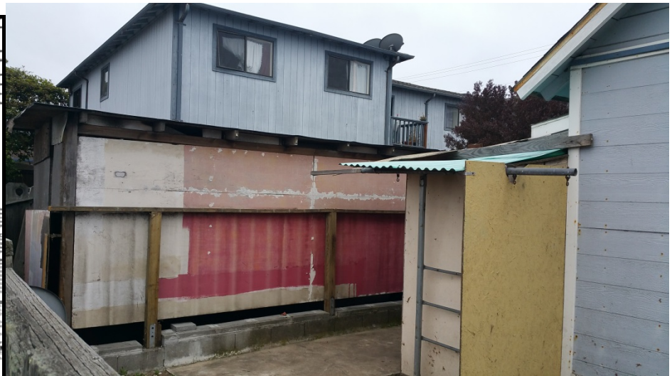
Existing garage structure (to be removed)
