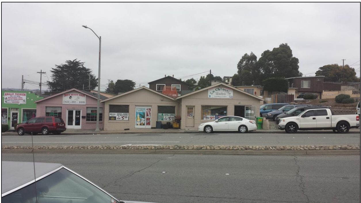
1482 Fremont from the west showing netting for condenser enclosure
