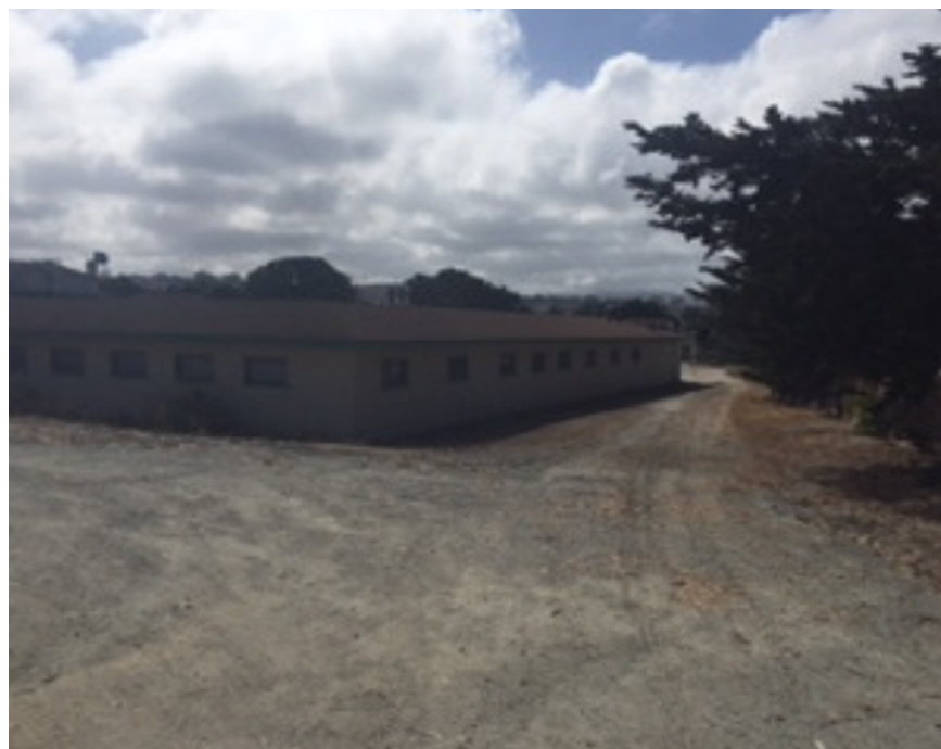
View of Classroom Building from northwest corner
