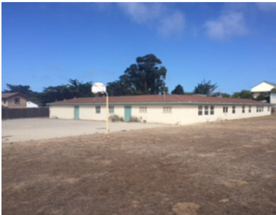
View of Classroom Building from Southeast corner
