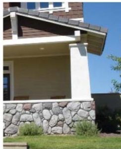
Walls of brick, siding, stucco, or stone
