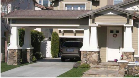
Horizontal emphasis of building forms
