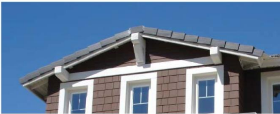
Decorative beams and braces below gables
