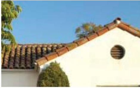
Red barrel tile roof
