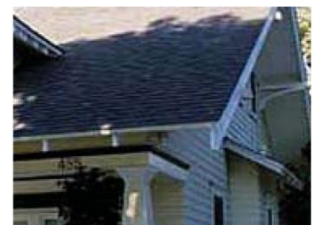
Flat tile roof
