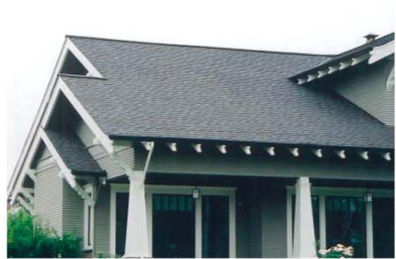
Exposed rafter tails
