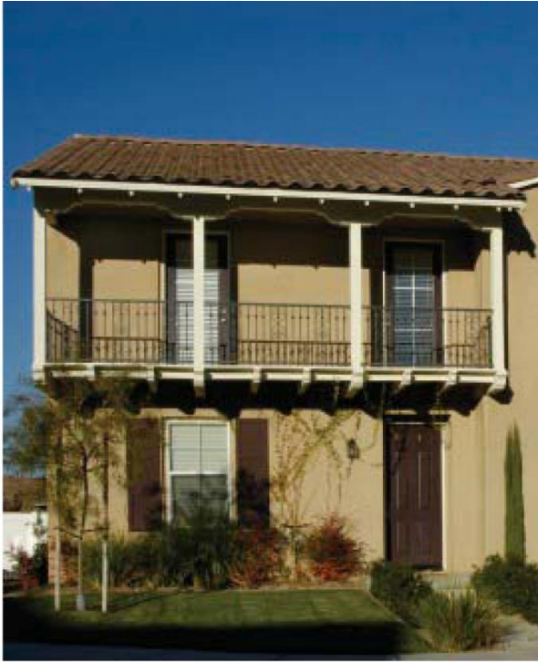
Cantilevered balconies along front facade
