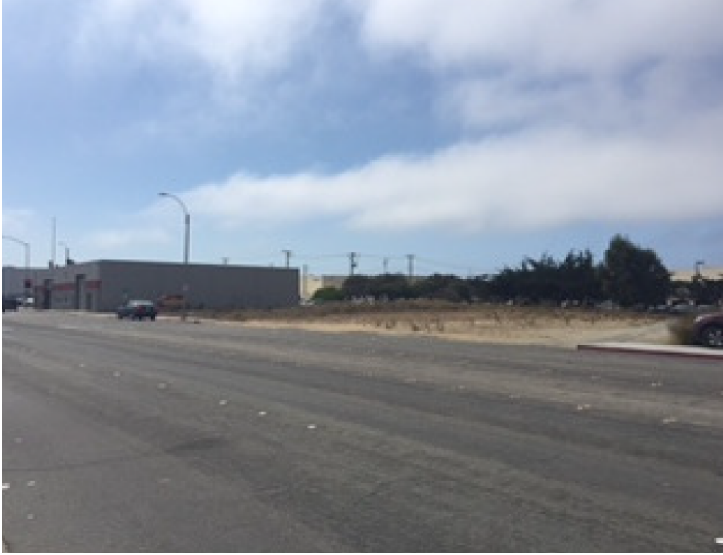
View of northeast corner of the proposed parking lot and north elevation of the existing building
