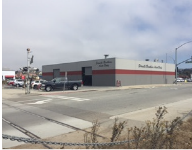
View of Rear (West) Elevation
