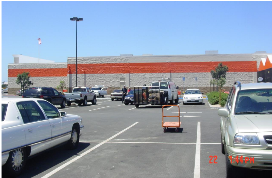
View of "Christmas Tree" Sales Area from Rear Parking Lot Looking West
