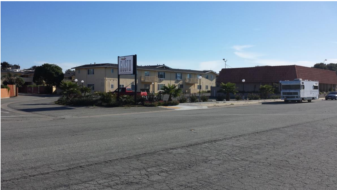
View of site from S side of La Salle Avenue looking towards restaurant and parking lot.
