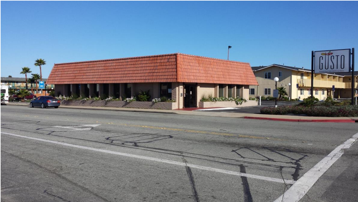
View of site from SW corner of Fremont Boulevard and La Salle Avenue.
