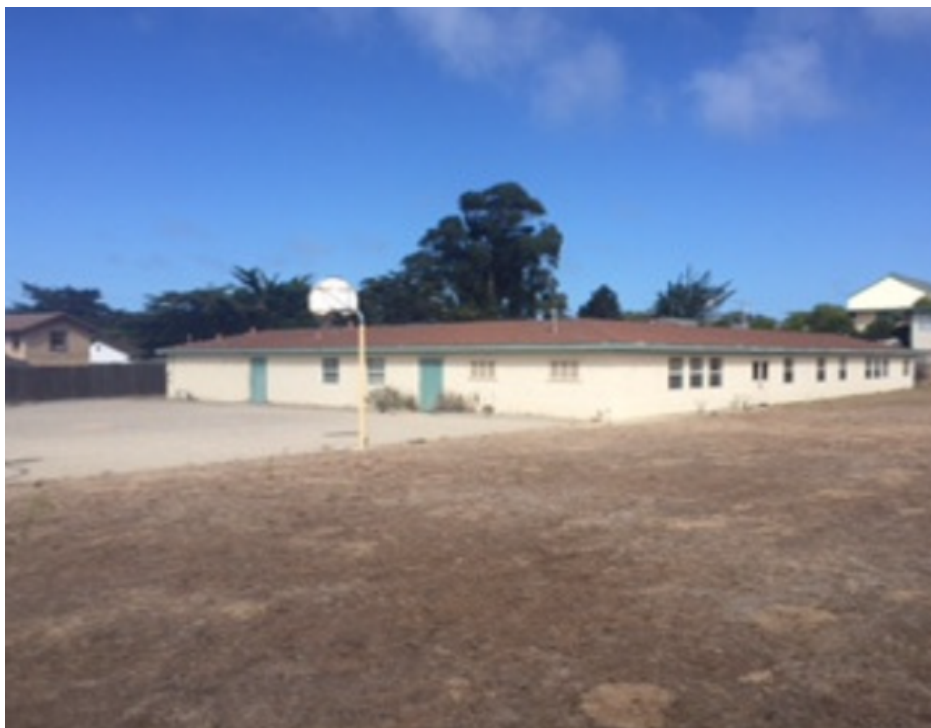
View of Classroom Building from Southeast corner
