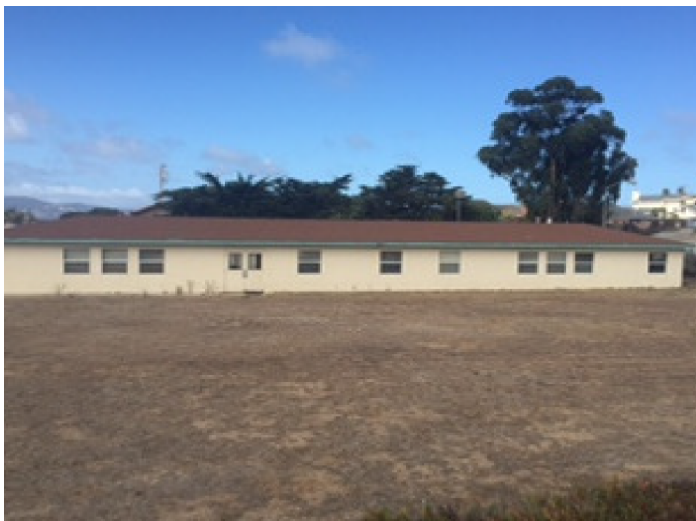
View of Classroom building from east side
