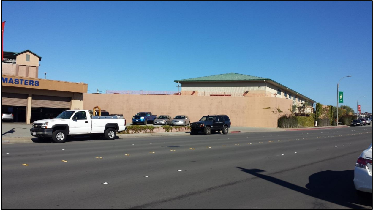
Street View from Del Monte Boulevard showing netting
