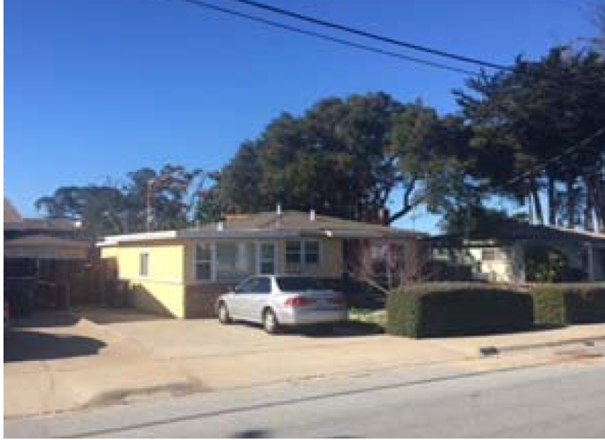
Street View looking north
