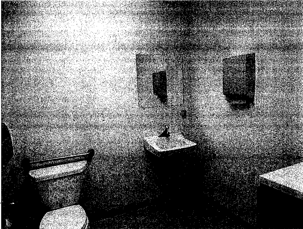
BUILDING B TYPICAL RESTROOM
