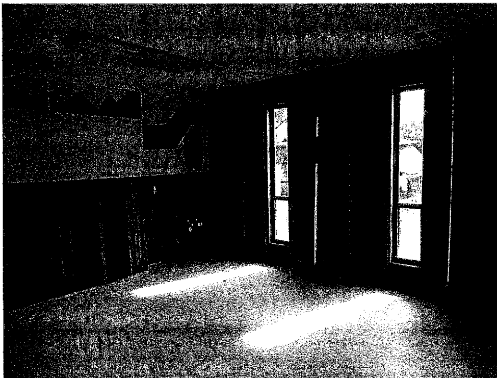
BUILDING B OFFICE WHERE SHEETROCK WAS REMOVED DUE TO FLOODING
