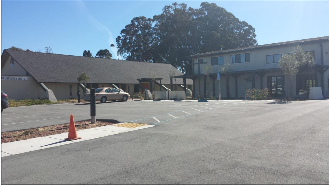
Parking Lot, Church, and Community Center from Driveway
