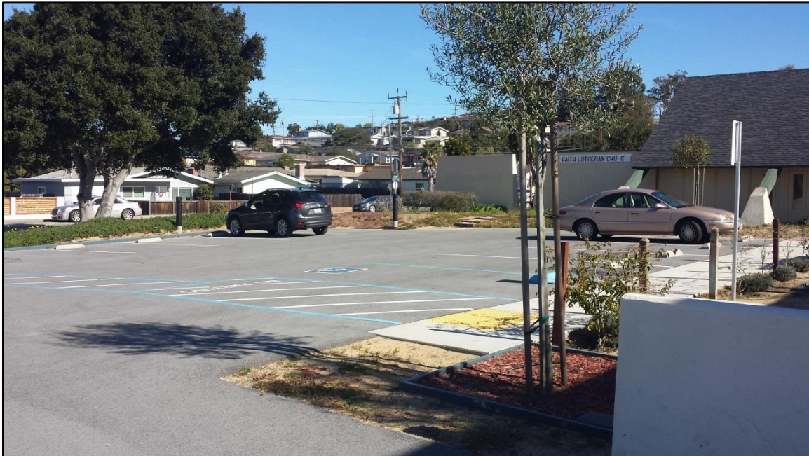
Parking Lot looking from West End of Community Center
