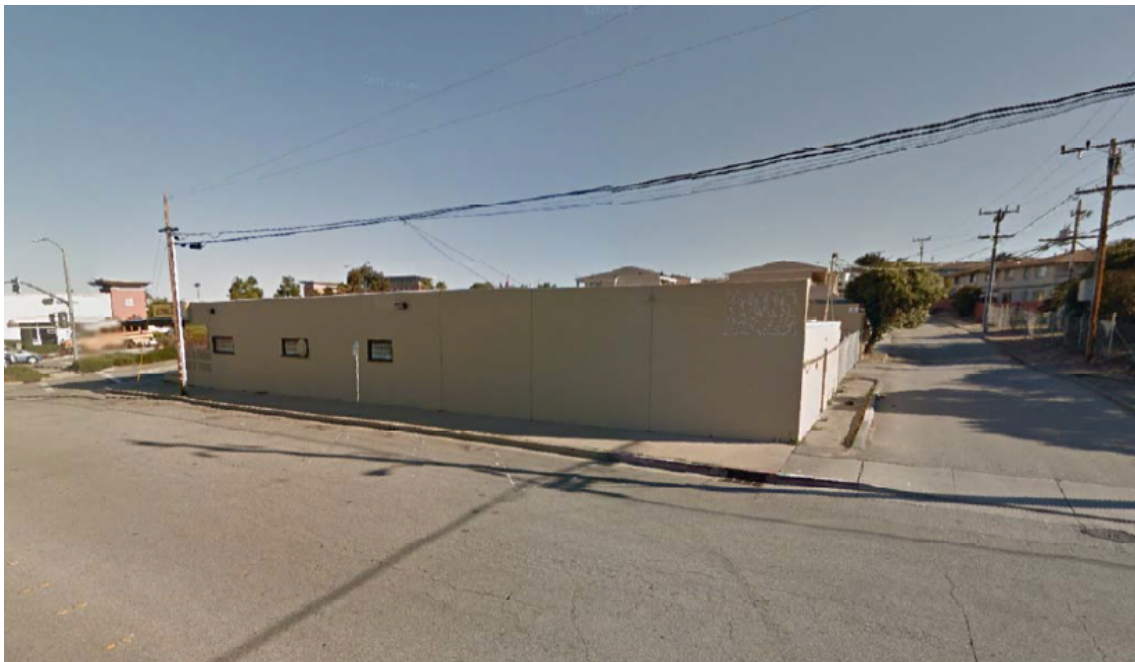
View of south side facing Playa Avenue
