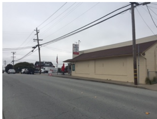
View of Front Building Façade from Noche Buena Street looking north
