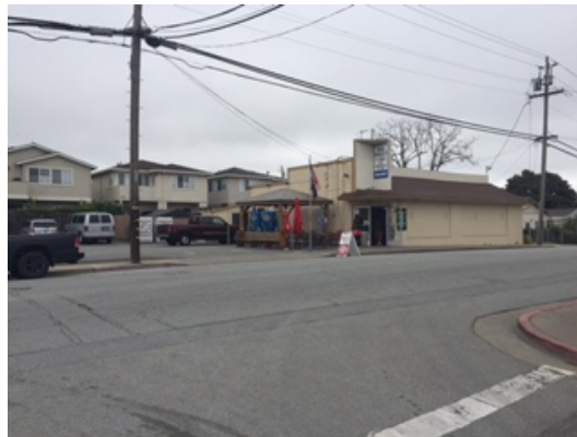
View of North Building Elevation and covered seating areas from Noche Buena Street Looking east
