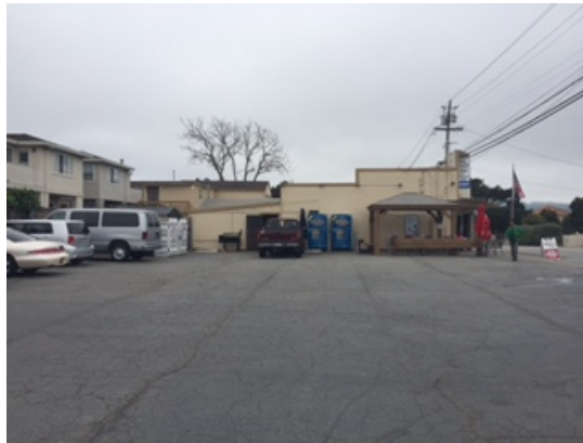
View of North Building Elevation and parking Lot from Wanda Avenue looking south
