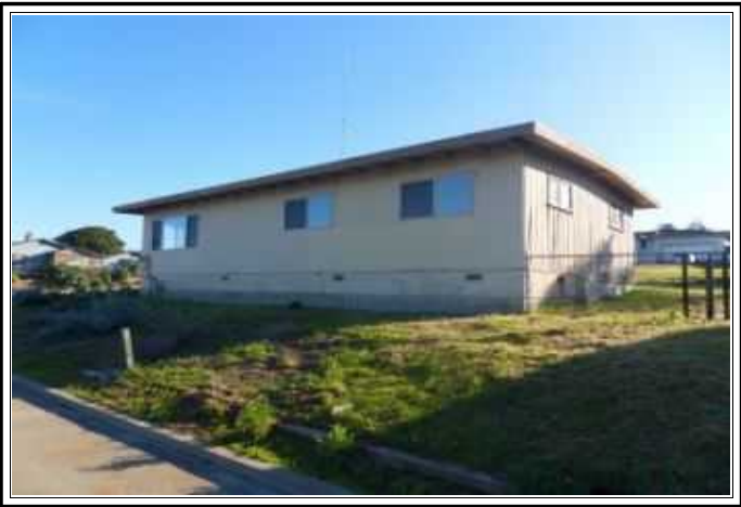
side view from street
