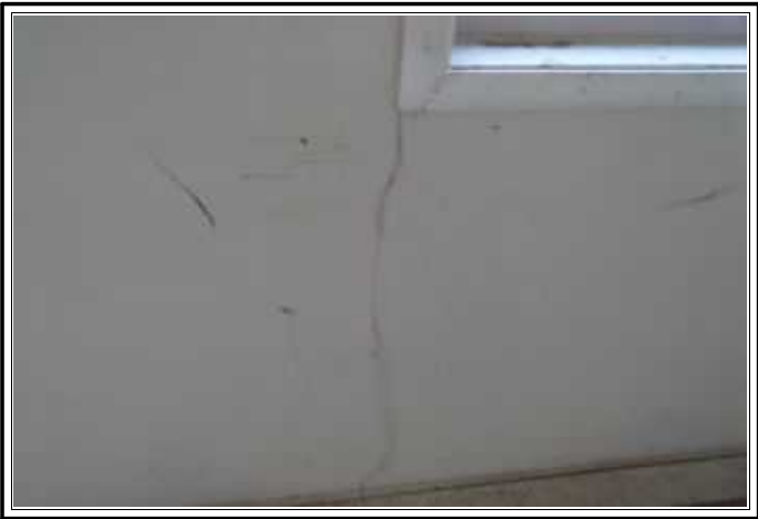
damaged sheetrock
