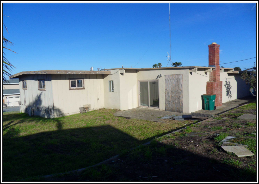
REAR OF SUBJECT PROPERTY
