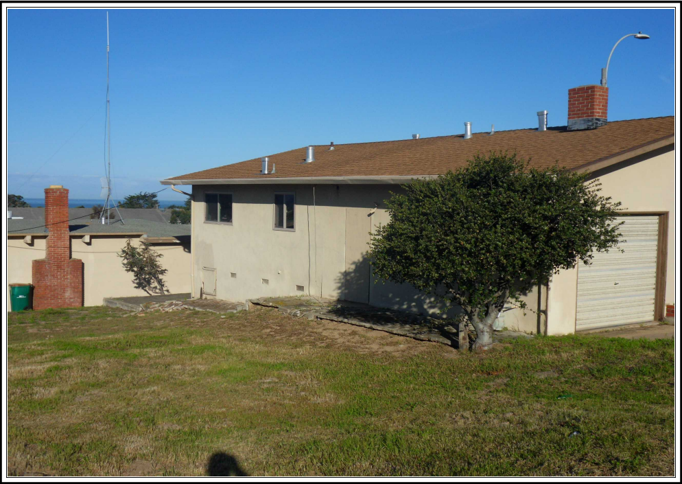
REAR OF SUBJECT PROPERTY
