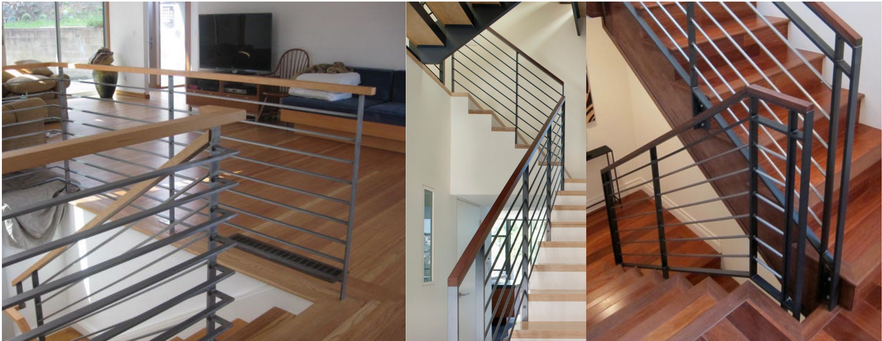
Railing Metal railing with wood handrail
