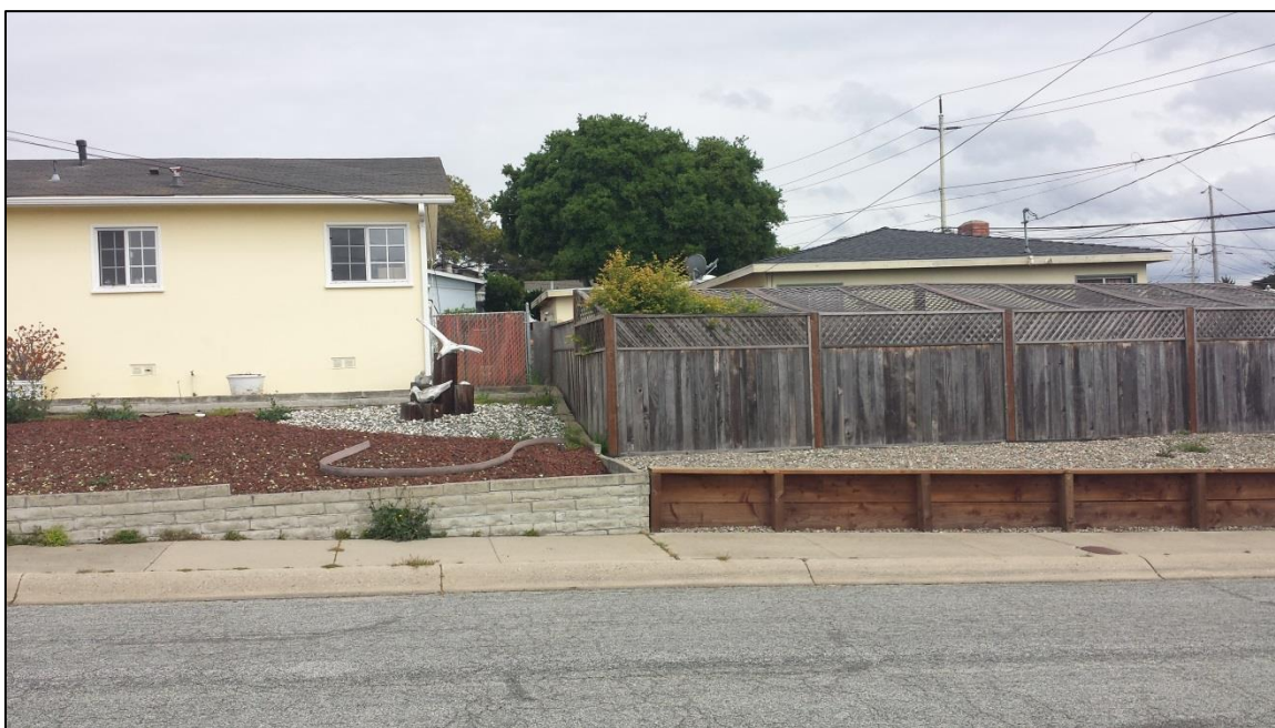
West end of house from Madera Court
