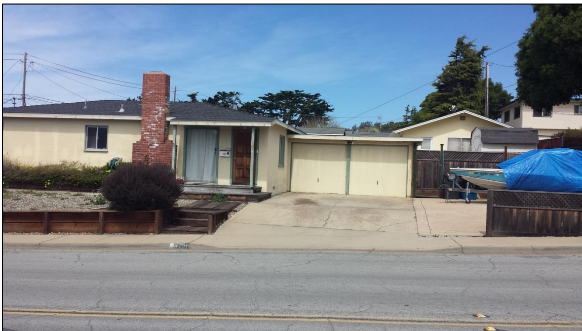
Existing two car garage from Kimball Avenue
