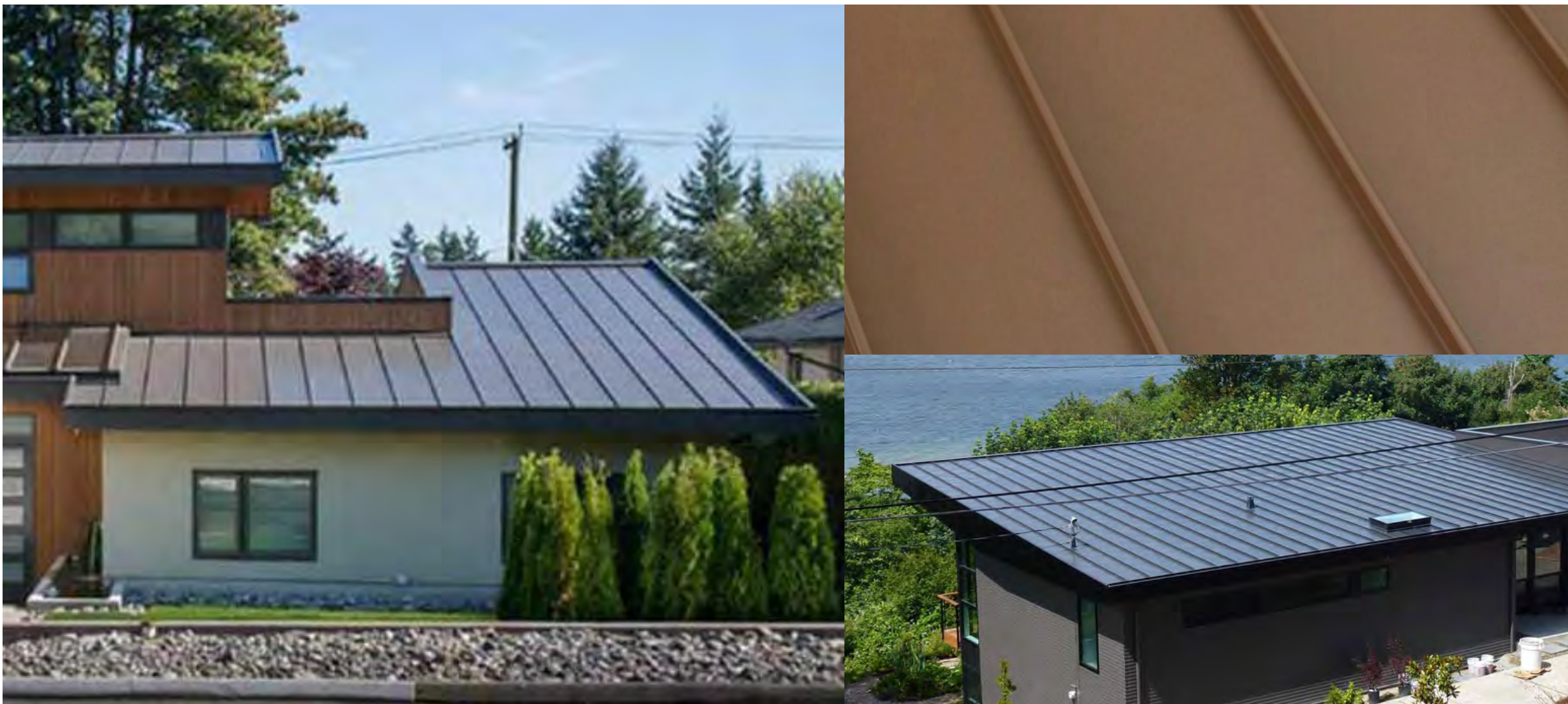
Roofs Standing Seam Metal Roof Dark Brown
