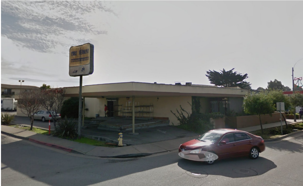
View of northwest corner of storefront from Fremont Boulevard
