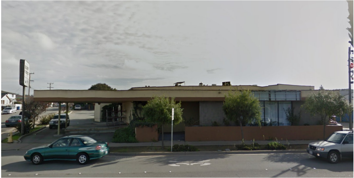
View of Front Façade from Fremont Boulevard looking East
