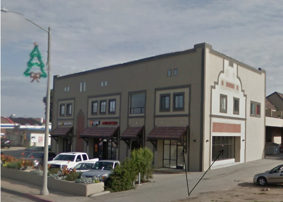
View tenant space at southwest corner from Fremont Boulevard
