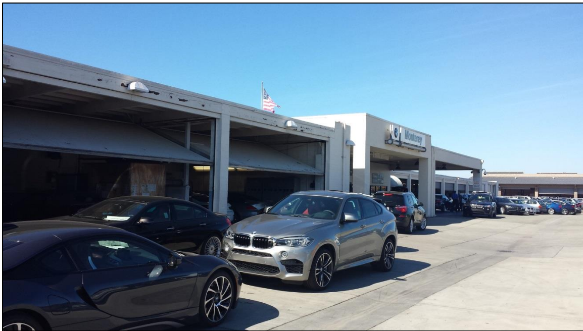
View of Service Area from southeast corner of property
