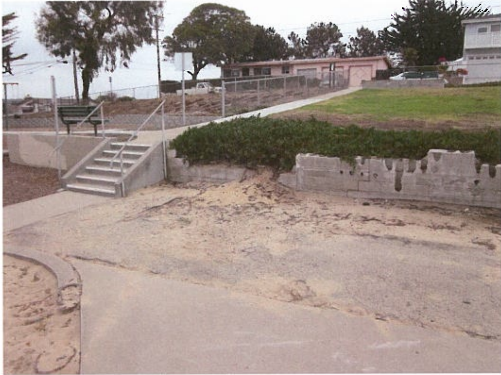
Condition of Retaining Wall
