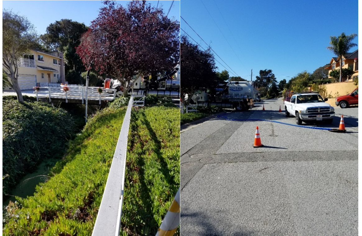
Vactor pump set at about 230 ft. downstream of the sewer main break to pump contaminated water from the creek into the sewer.
