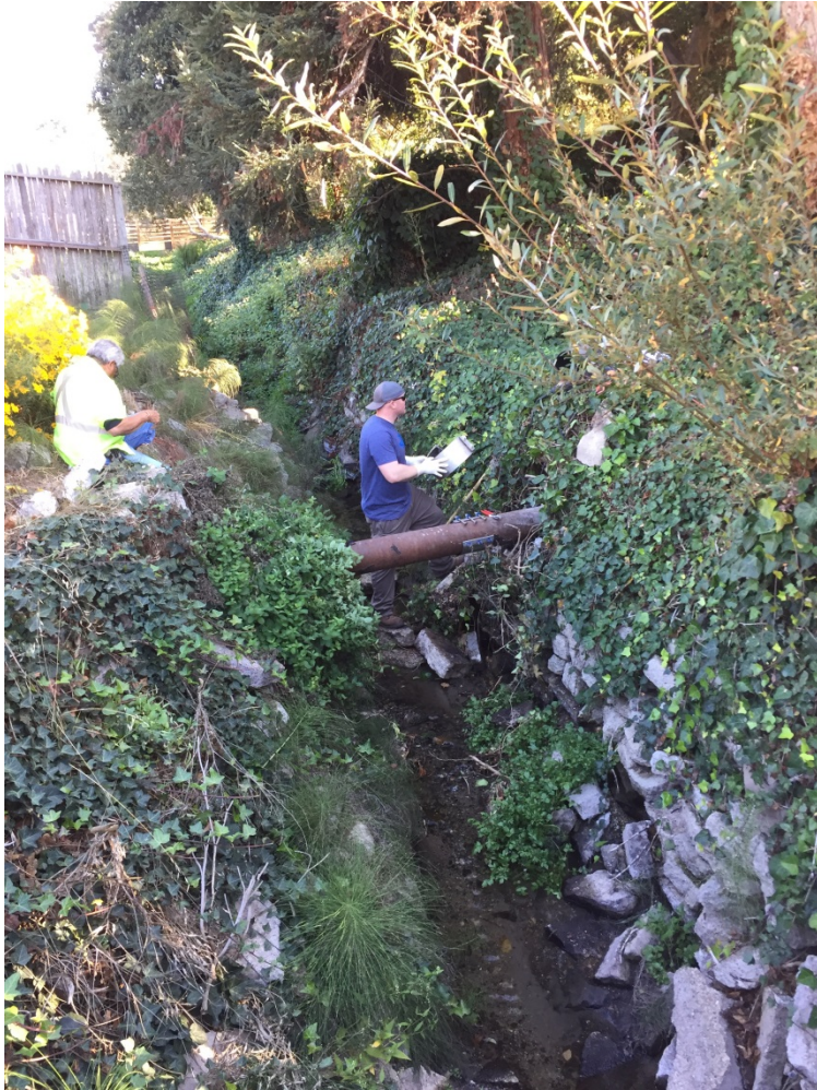
External band clamps and patch materials being installed on the pipe crossing the creek.
