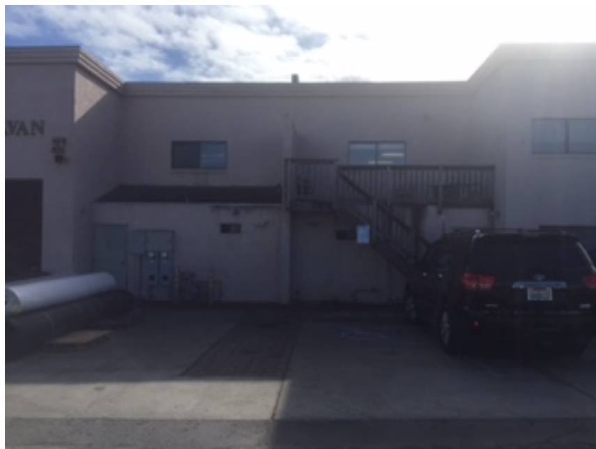
Rear Façade from alley
