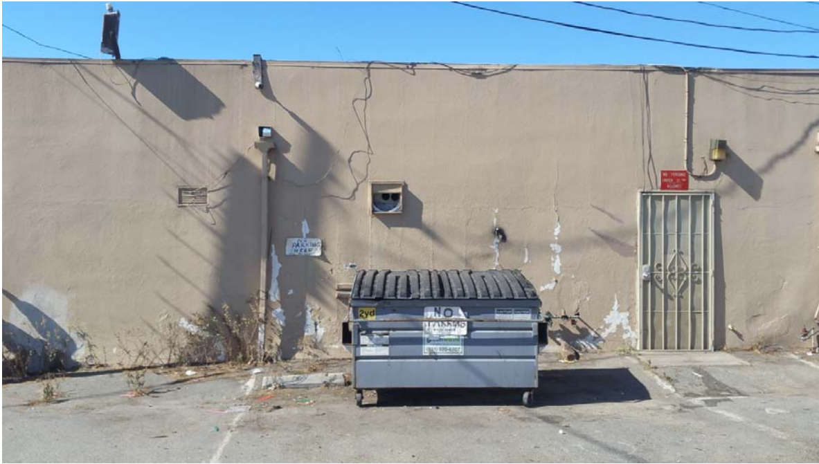
Figure 3. Existing back of building, picture taken from alleyway facing West.
