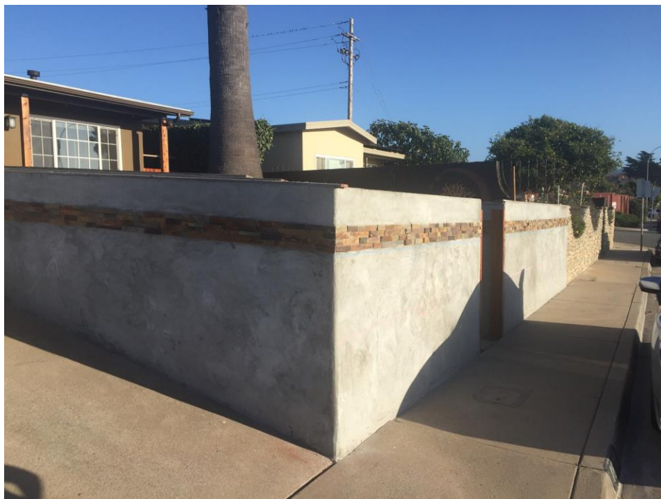
View of wall looking south on the sidewalk
