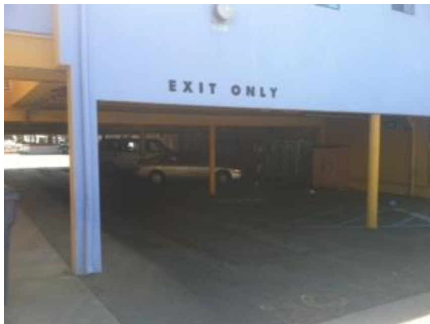
View of parking area under 1123 Fremont Boulevard
