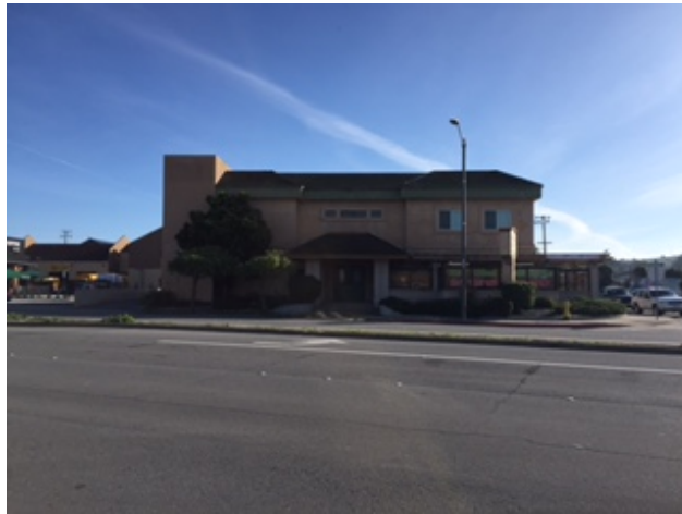
View of Front Façade from Fremont Boulevard
