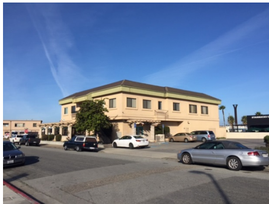
View of rear elevation and Parking Lot
