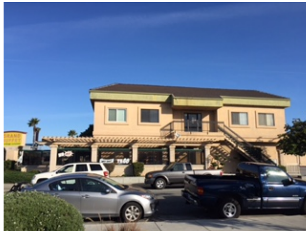
View of Street Side elevation from Birch Street
