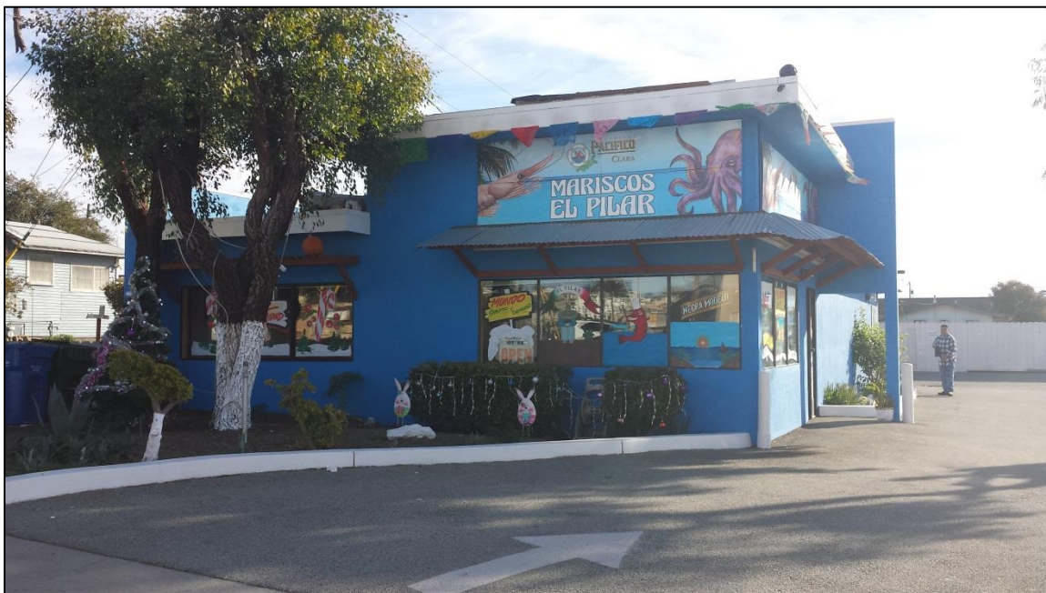
View of front of restaurant from La Salle Avenue
