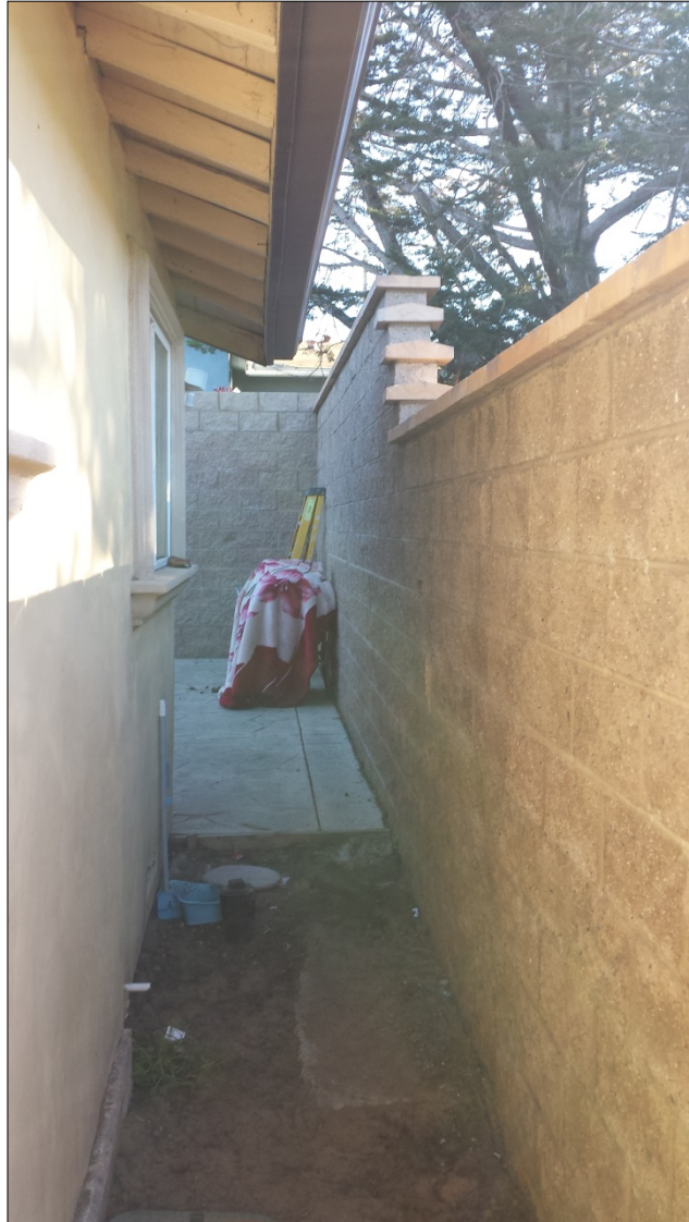
View of side yard towards rear of property
