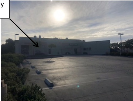
View of rear façade facing parking lot
