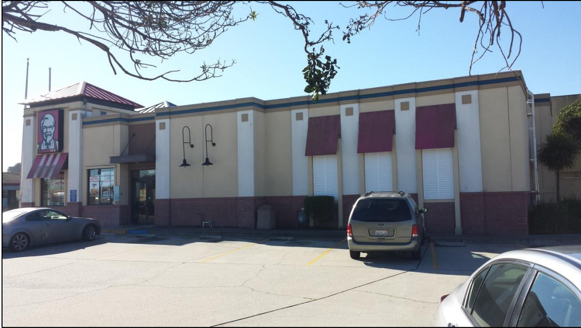
View from Hilby Avenue
