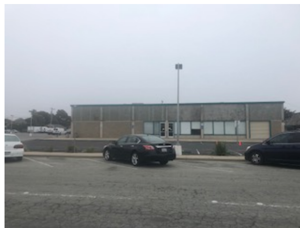
View of east side elevation
