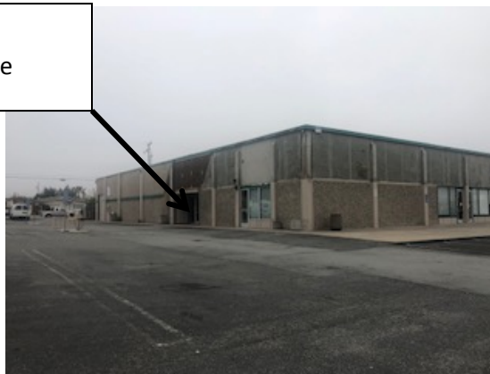
View of Front and north side elevation
