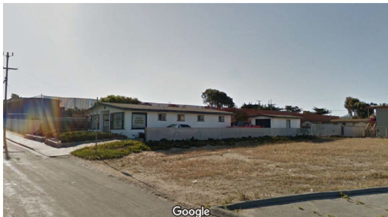
View of west side from Playa Avenue
