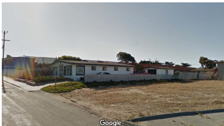
View of west side from Playa Avenue
