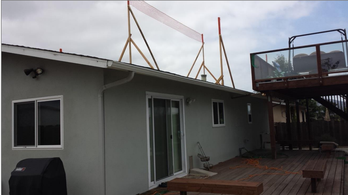
Side of house showing existing deck and flagging for addition
