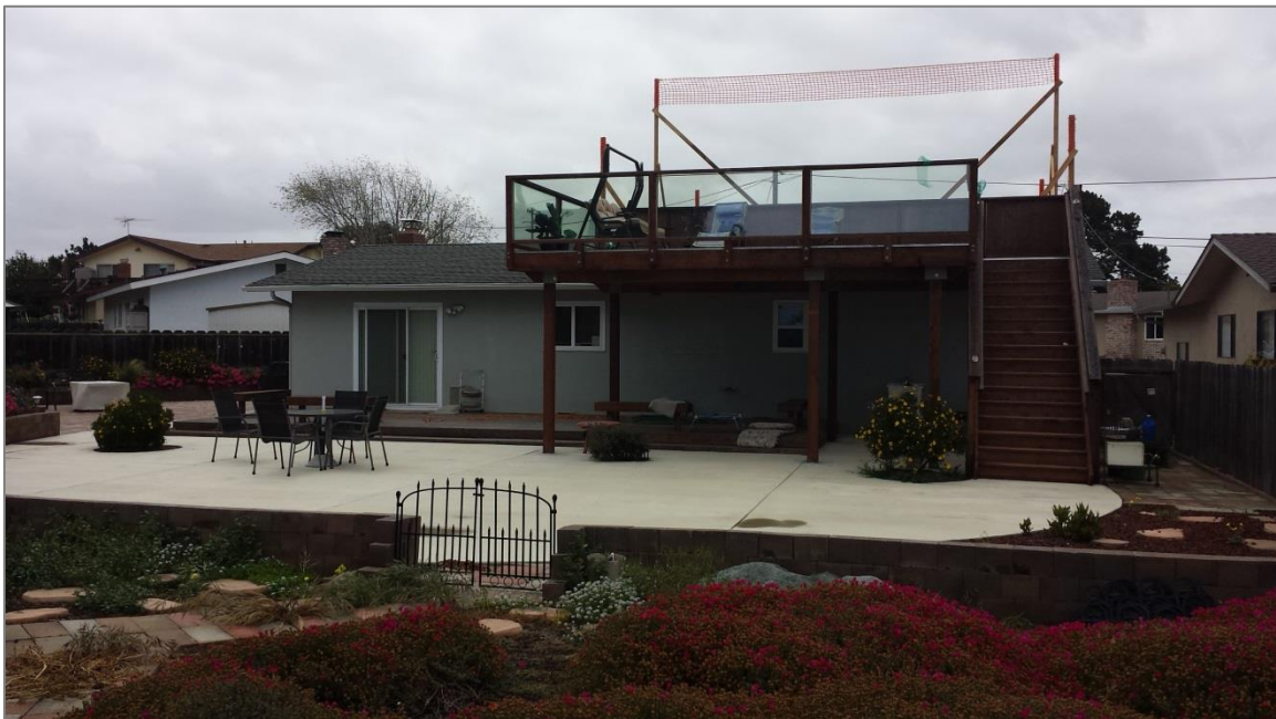
Rear of house showing existing deck and flagging for addition
