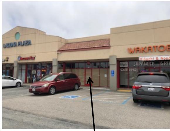
Front Façade looking east
