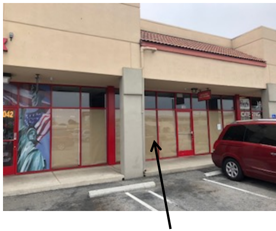
Front Façade looking west
