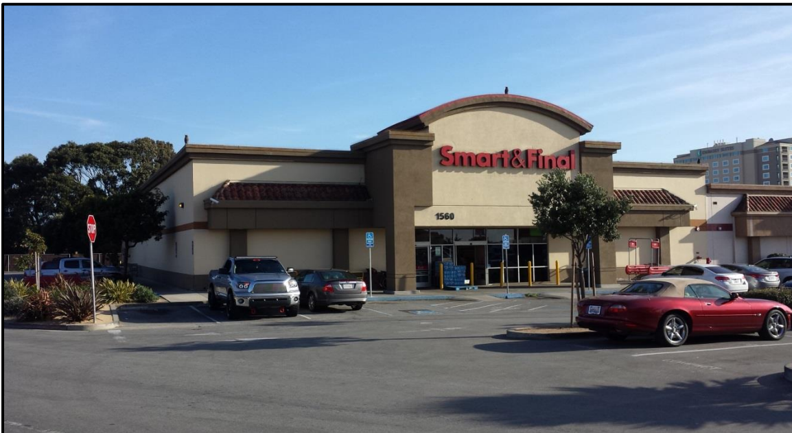
Front and North elevation from the parking lot
