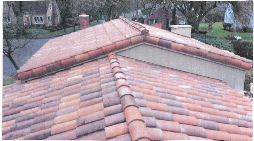
SPANISH CLAY TILE ROOFING
