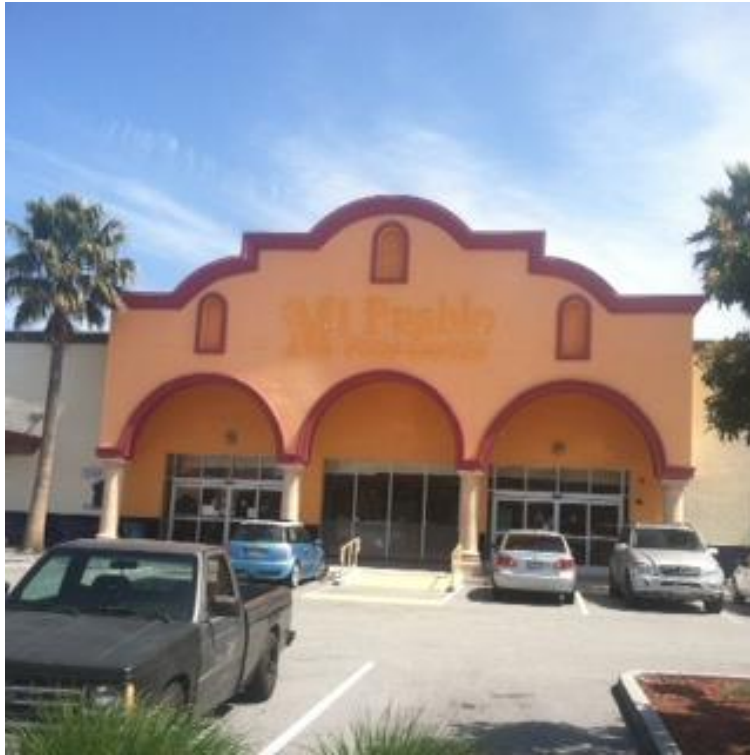
View of portico projection facing parking lot on southern frontage
