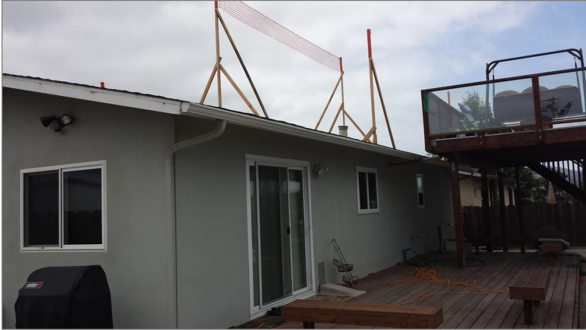
Side of house showing existing deck and flagging for addition
