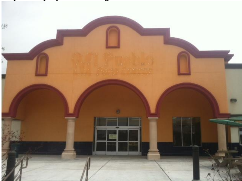
View of portico projection facing Fremont Boulevard on western frontage
