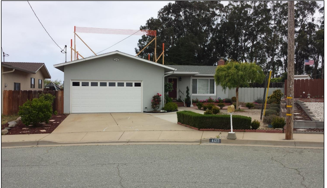
Front of house showing flagging
