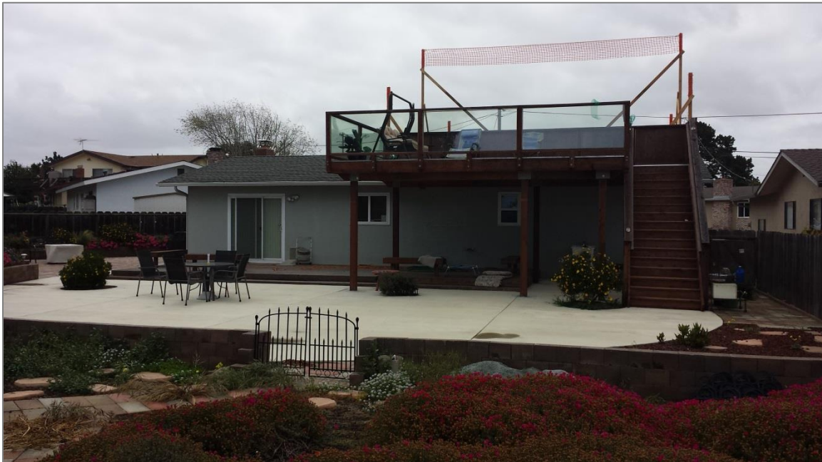
Rear of house showing existing deck and flagging for addition
