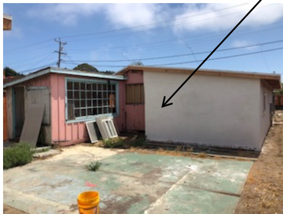
West Side of rear elevation
