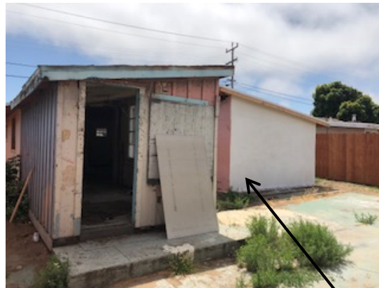
East side of rear elevation
