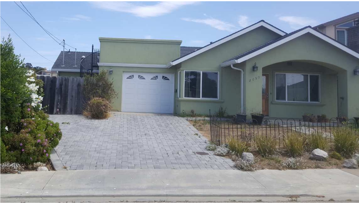
FRONT VIEW - WITH STAIR INSTALLED
