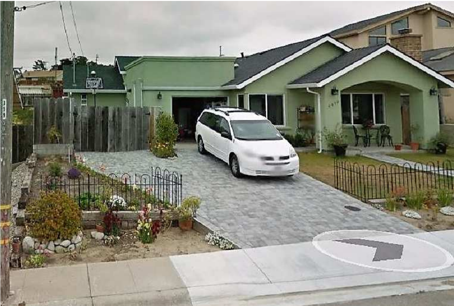
FRONT VIEW - PRIOR TO STAIR INSTALLATION GOGGLE MAPS
