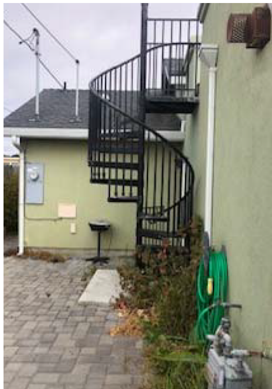
View of Spiral Staircase
