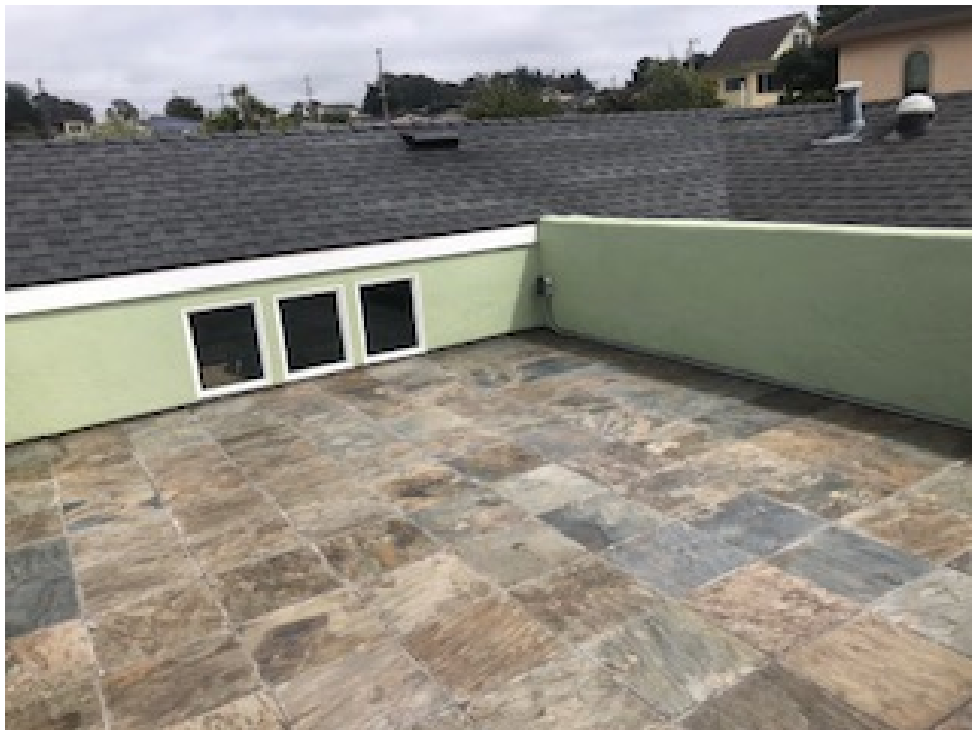
View of roof deck looking to the east
