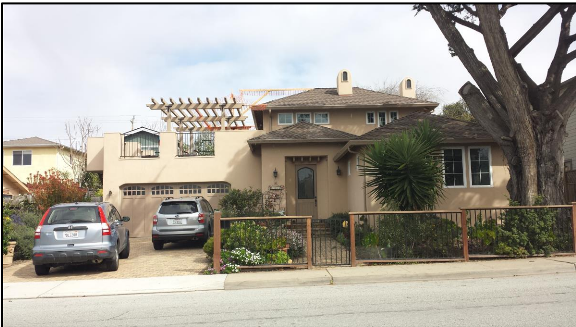
View of front of house from end of Palm Avenue showing flagging
