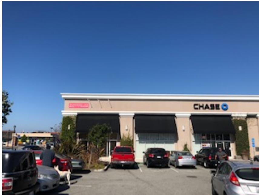
Front façade from interior parking lot
