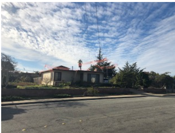
View of Front Façade looking Southwest
