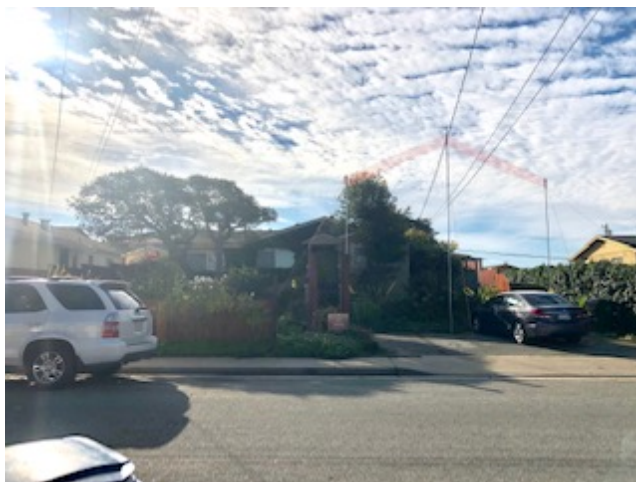
View of front façade looking south
