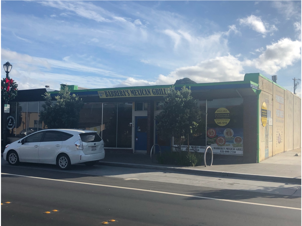
View of front facade
