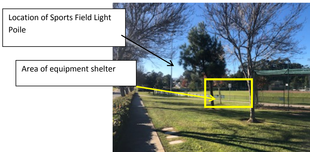
View of Sports Field Light Pole and equipment enclosure
