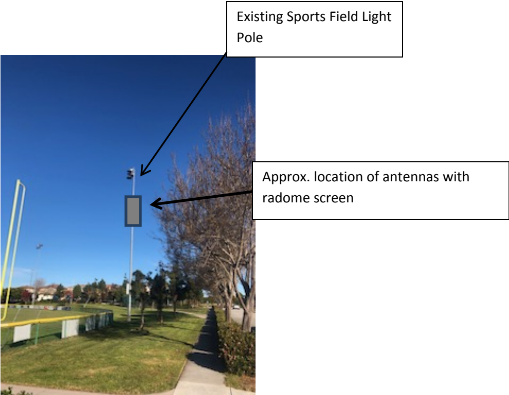
View looking North
