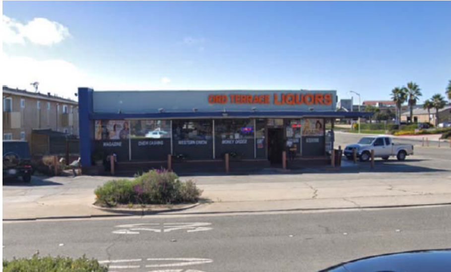
View of the front façade for Liquor Store
